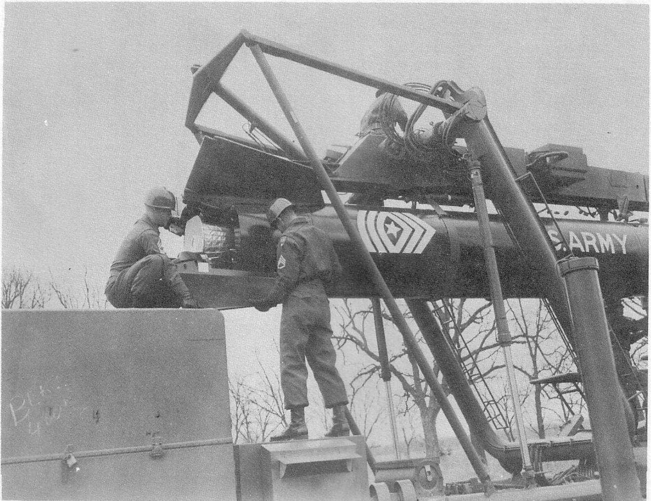
Figure 14. Control surface attachment.
